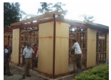
The new office extension building construction
