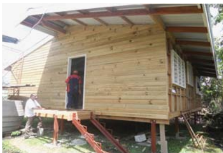
New Goroka transit house, still under construction
